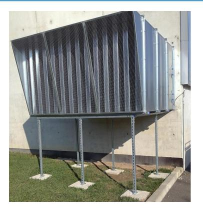
The noise emissions by the Rosny plant were higher than the limit fixed the regulations. During joint inspections by dB Vib Consulting our teams identified the main sources and imagined treatment solutions to reduce the emissions below the regulation levels. This type of organisation allows us to combine good technical knowledge and acoustic expertise to match the solution to the goals fixed by the inspecting bodies.
