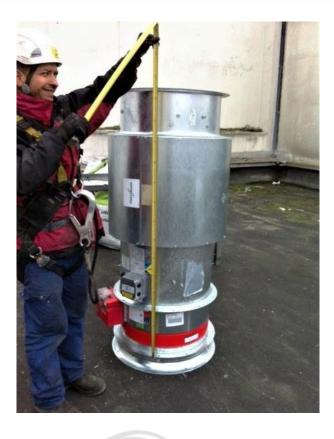
ENEDIS, with the support of its service dedicated to source substations (BRIPS), has selected dB Vib Ingénierie to **perform the replacement of the ventilation system** in Turgot source substation (18e arr). This project is part of a large campaign for retro-fitting the intra muros parisian power substations.
