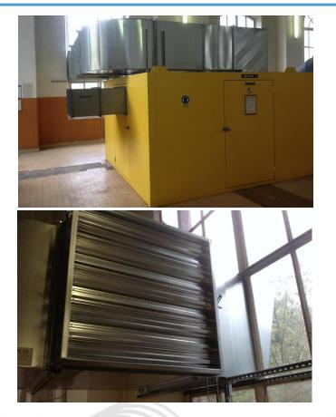
The group 1 of the SAUVIAT plant owns an acoustic enclosure that dates from the creation of the plant. There were overheating issues and it was necessary to **upgrade the ventilation system** of the groups.
