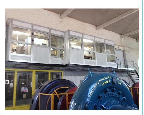
Willing to improve the staff working conditions, the GEH from TARN had placed a call for tender to define an acoustical treatment solution to **reduce noise on a monitoring platform** in an hydroelectric power plant.
