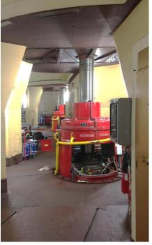
The Electricity Power Station from PEYRAT LE CHÂTEAU has a configuration quite exceptional since it is at **60 m underground**, with an access via a long access and maintenance tunnel.
