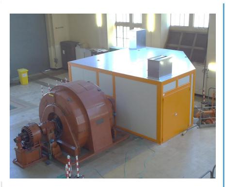
The GEH from LOIRE-ARDECHE has consulted with dB Vib to perform **an acoustical audit on the turbine** 5 of the Monistrol d'Allier power station.
