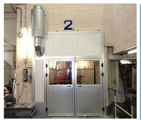
The Marcillac plant is part of the Chastang hydroelectric power station and comprises 2 generators. As Generator 1 was entering a long period of maintenance and renovation, EDF wanted to **treat Generator 2 acoustically** in order to allow operators working in the plant to do so in sufficient **comfort**.
