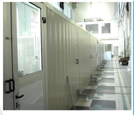
In 2010, the 4 generating units of the VAL BEYNETTE power station had successively been in maintenance. So the GEH launched an invitation to tender to **design and realize acoustical treatments** allowing to work in maintenance on an hydraulic power unit while the other ones are operating.
