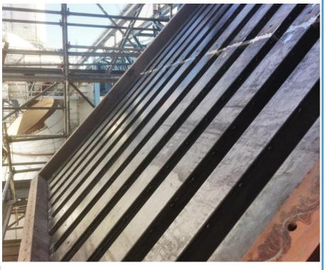
After the installation of a filter on a smoke treatment line, the existing silencer no longer sufficed to achieve the objectives of noise emissions in the vicinity.
