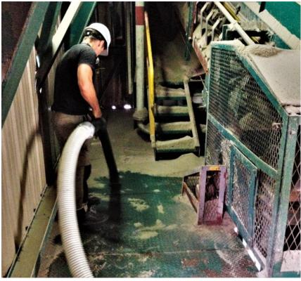
ALBIOMA, on the BOIS ROUGE site on Réunion Island recycles the sugarcane wastes (bagasse), to produce energy. **dB Vib Ingénierie** has intervened to **design and install an high power central vacuum suction system** (NCV) (vacuum unit 30KW).
